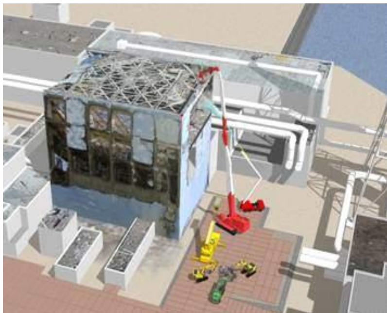
Removal of Rubble
