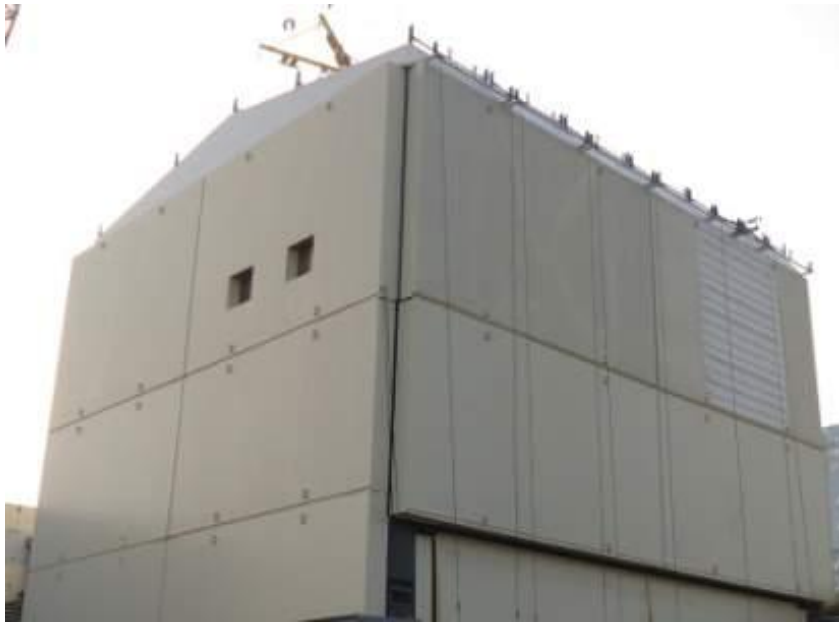
Reactor building cover installed on 1F Unit 1
