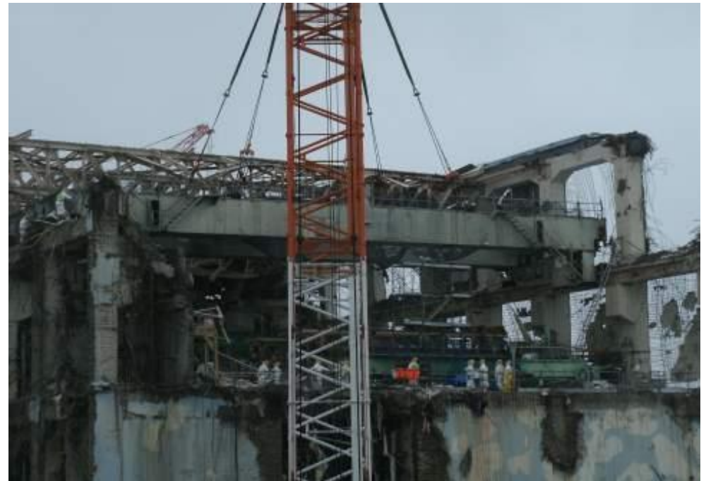
Removing rubble from 1F Unit 4
