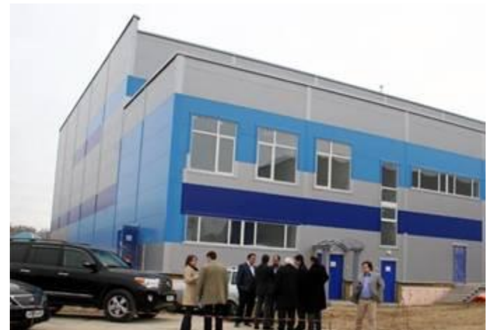
Radiation technology medical plant
