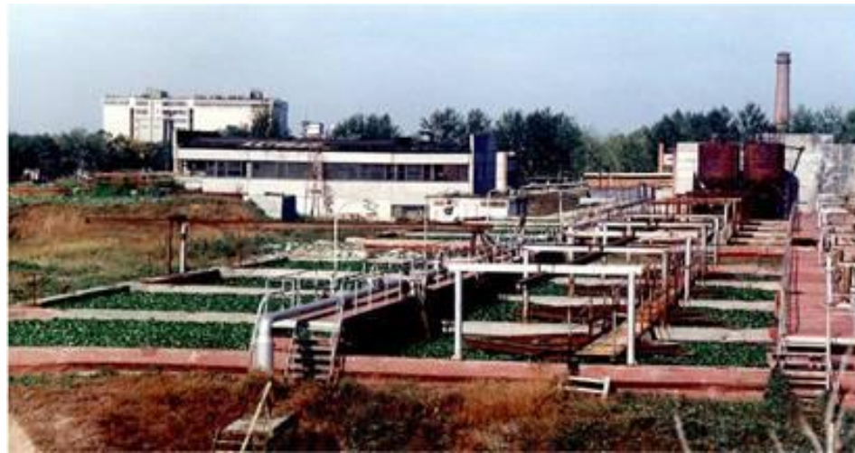
Kudriashi livestock waste cleaning facility
