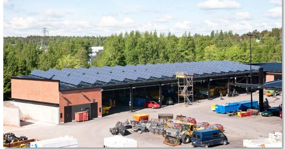
Espoo City car depot, a 55 kW PV system to charge electric vehicles – Helsinki Capital Area Climate Award 2011
