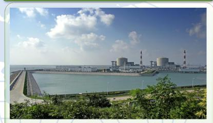
Units № 1 and 2 with VVER-1000/428 reactors having electrical capacity of 1060MW were put into commercial operation in 17.05.2007 and 16.08.2007, respectively.
