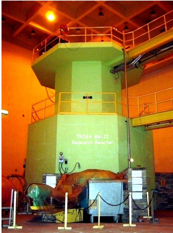
Shield Structure of the TRIGA Reactor
