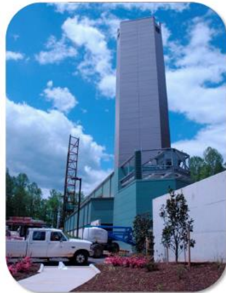
mPower: Integrated Systems Test (IST) facility (1:1 in height and P, T; 1:375 in power)
