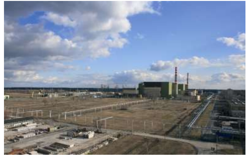
Site of the new units
