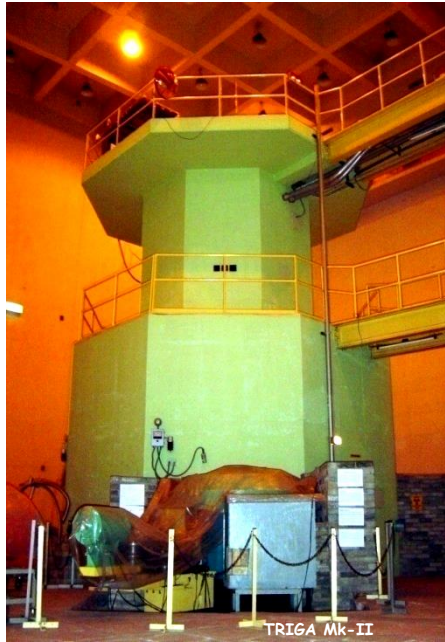
Shield Structure of the TRIGA Reactor
