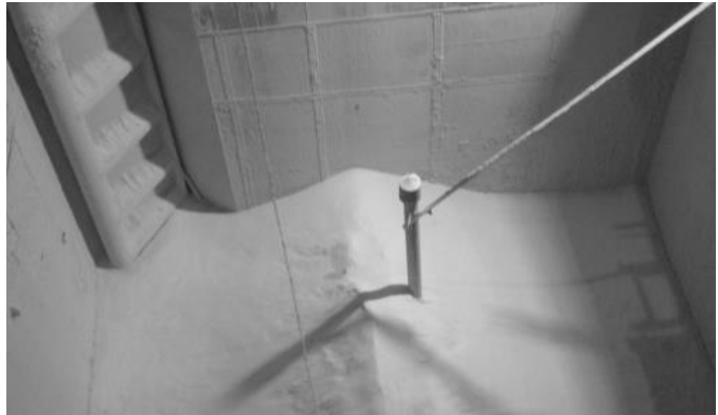
Control channel in technological area
