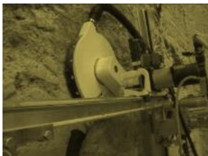
Decontamination of the central hall walls
