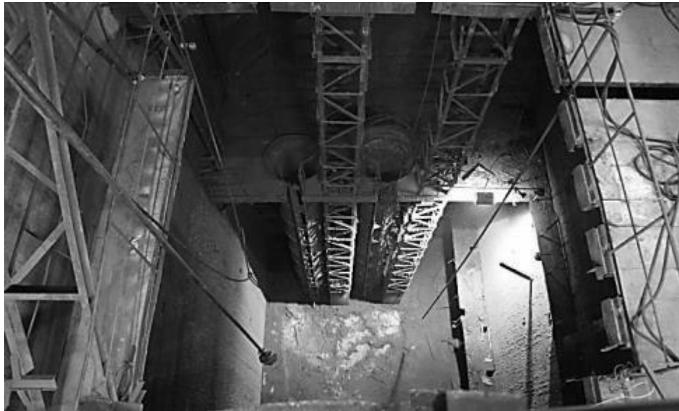
First stage of metal constructions dismantling
