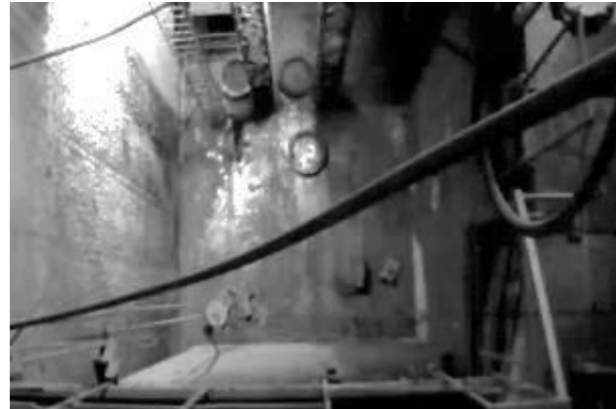
End stage of metal constructions dismantling
