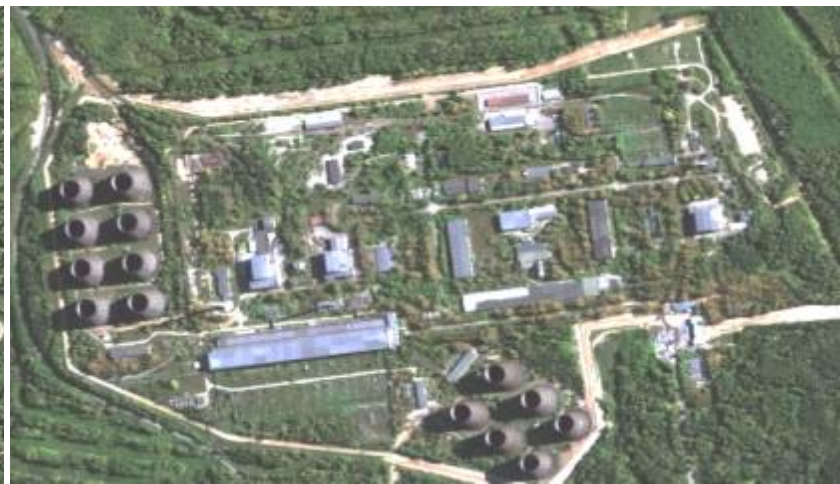
South site (area 2) - 3 industrial reactor plants
