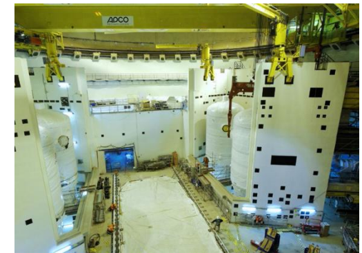
Reactor pressure vessel & 4 SGs introduced in the reactor building
