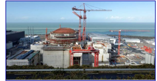
EPR construction at FLA3
