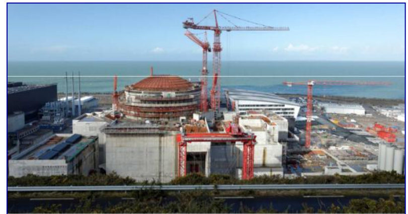
EPR construction at FLA3
