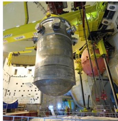
Reactor pressure vessel & 4 SGs introduced in the reactor building
