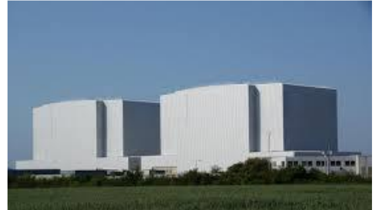
Bradwell Safestore - cladding complete
