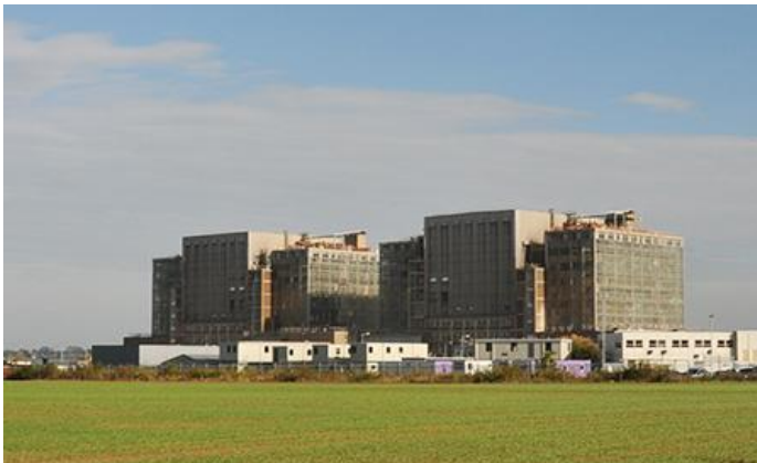
Bradwell Safestore - before cladding
