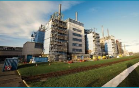
Harwell building demolitions
