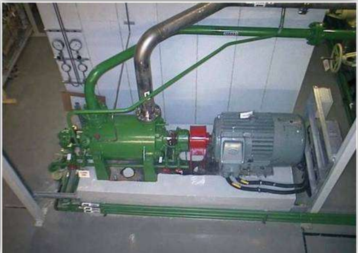
Relocation of the emergency feedwater system into a protected building
