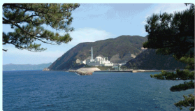
Fast Reactor Monju (to be decommissioned)
